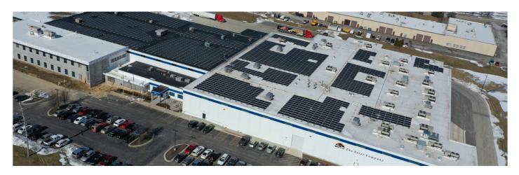
The system went live in February 2020 with an installed capacity of 675 kW. It is estimated to generate 810,000 kWh of renewable electricity per year. Over two years, the system has averaged 97.5% of its estimated performance.
